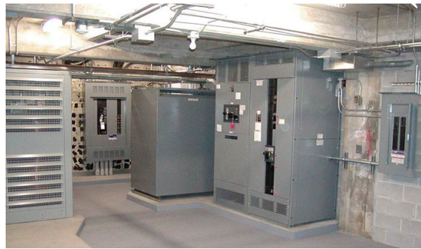
SWITCHBOARD DETAIL N.T.S. 1000A 277/480V 3PH, 4W 42,000 AIC
